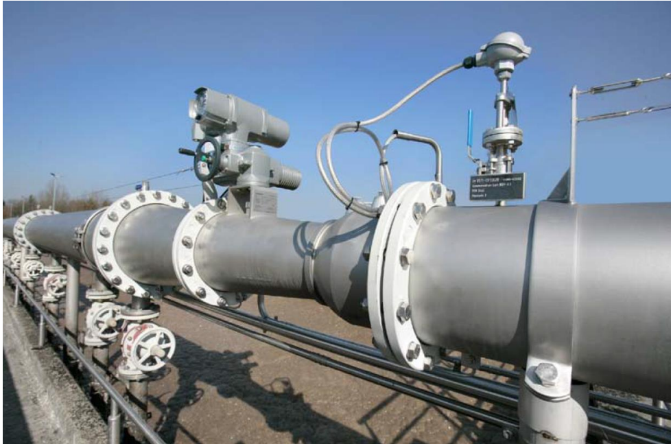
VACOMASS® jet control valve in a big German plant
